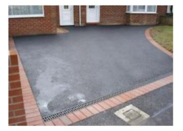
Example of a linear drain
