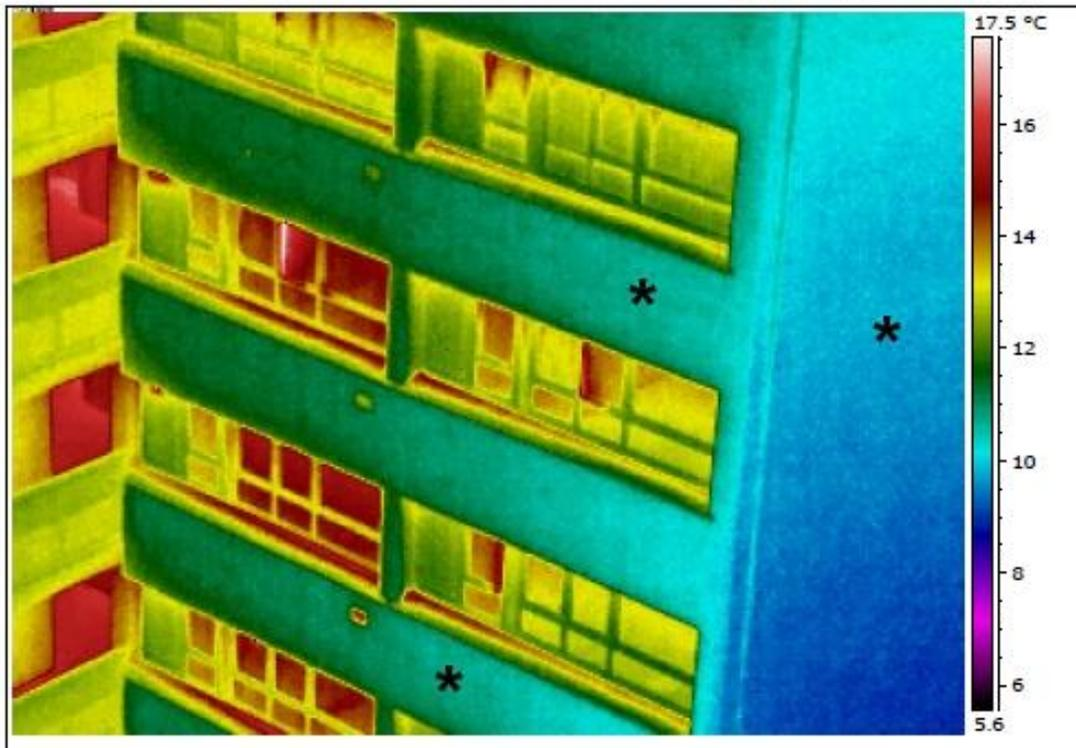
4, 5 and 6. Thermal image of elevation 7 (and 8) showing poorly defined thermal signature for barriers. Notably above slab level to elevation 7 as shown below.
