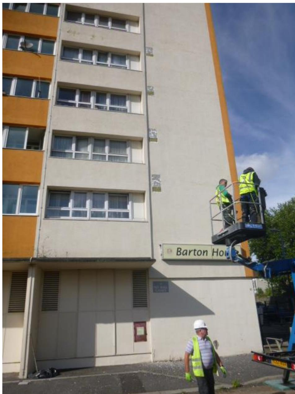
**8. Elevation 4 with fire barriers at each floor level around the stairwell enclosure.**
