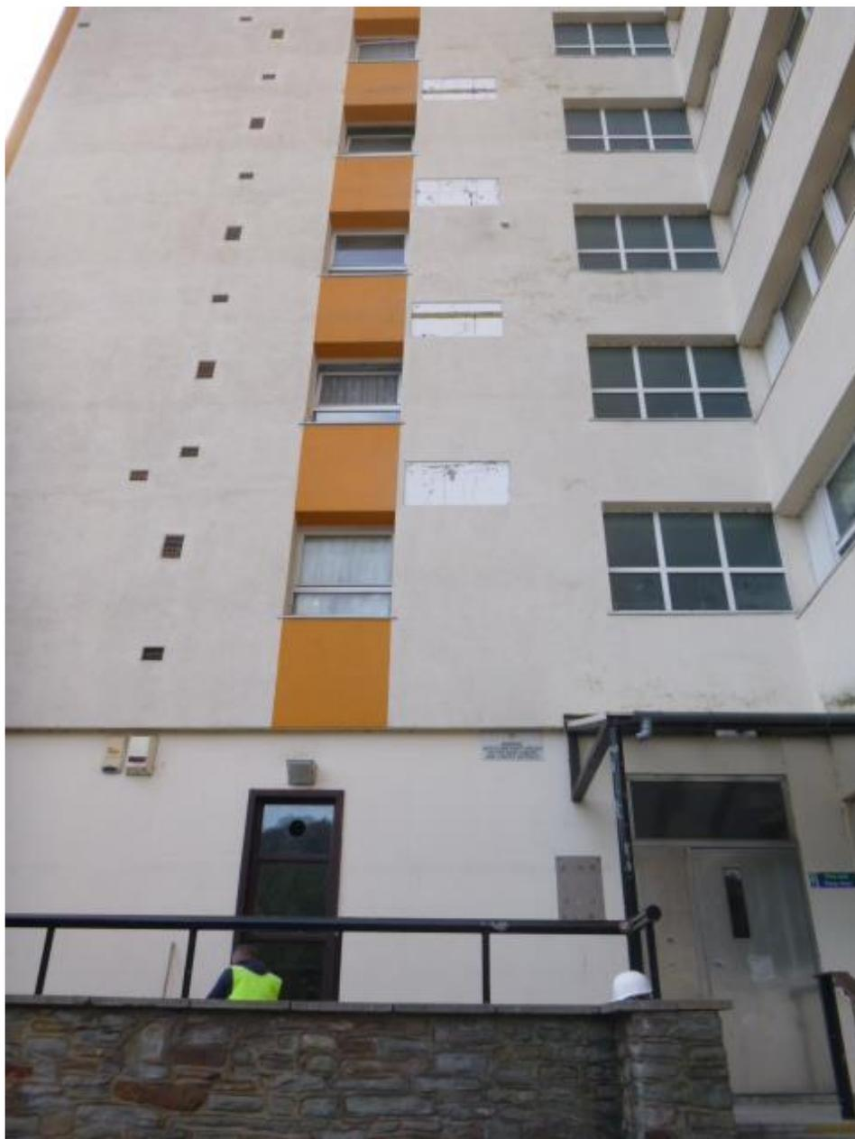
**7. Elevation 3 with fire barrier found at alternate levels from third floor upwards.**
