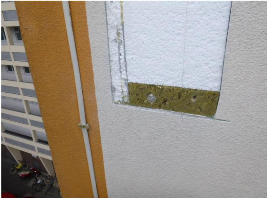
**11 Elevations 8 note fire barriers stop approximately 900mm short of the corner with elevation 7 and therefore would not be continuous even if installed at the same level**
