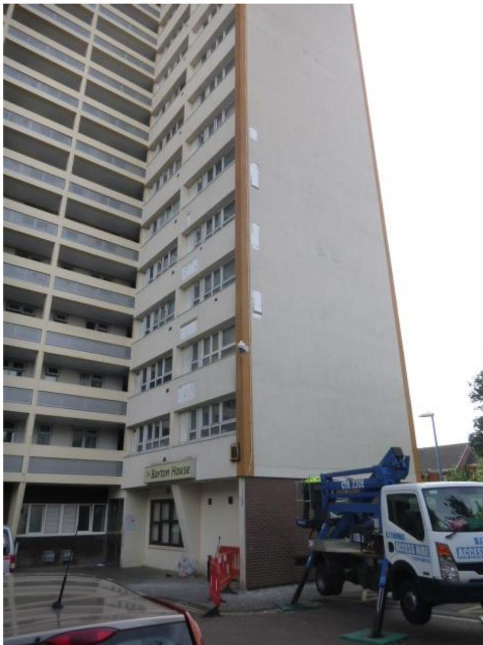
**10 Elevation 8 note fire barriers still at alternate levels but installed at slab level and therefore not continuous with elevation 7**
